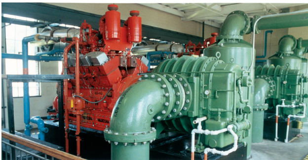
Roots' positive displacement blowers can be controlled with variable frequency drives to match air flow to process demands. The result is high process performance and low energy demand.
